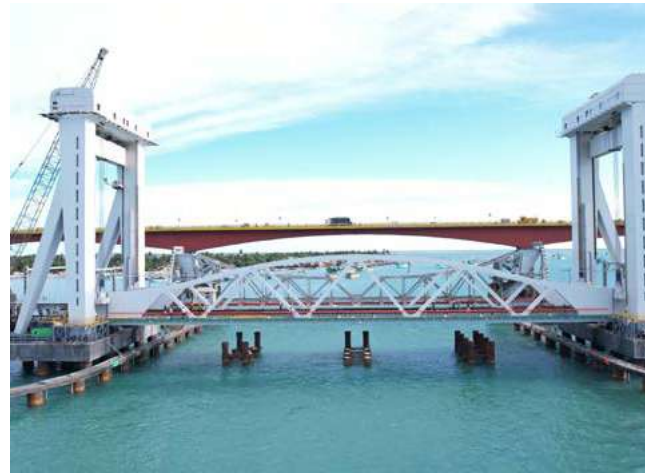
The Pamban Bridge, India's first vertical lift railway sea bridge
