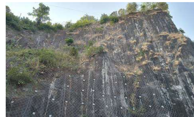
GALSTAR™ Wires installed at Mumbai's iconic Gilbert Hill
