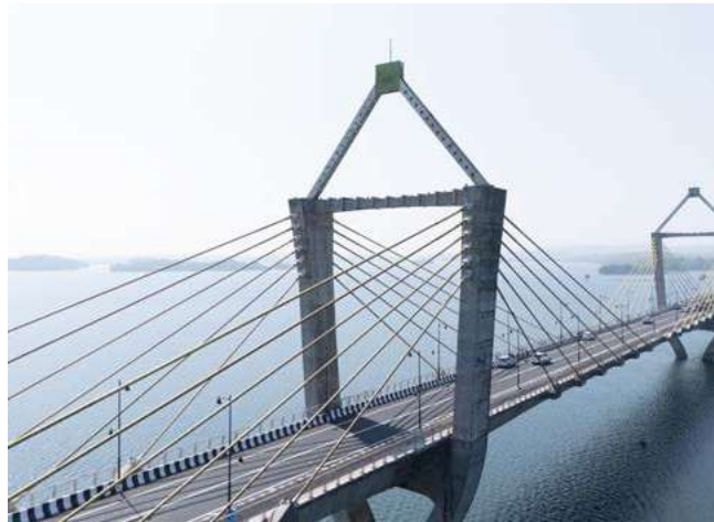
The Ambargodlu-Kalasavalli Bridge in Karnataka, India's second-longest cable-stayed bridge
