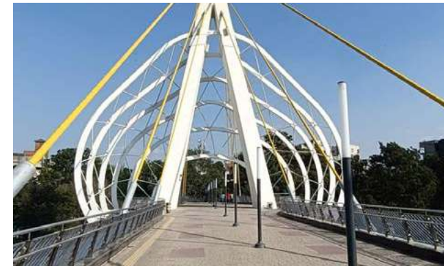
Pune city's longest flyover and the first cable-stayed pedestrian bridge across the Mutha River
