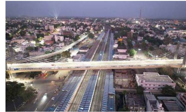
India's longest cable-stayed railway over bridge, Jabalpur
