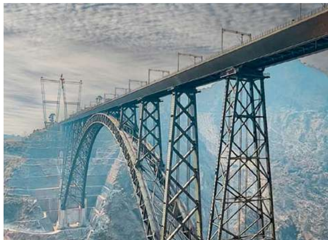
Chenab Bridge in Kashmir, the world's highest railway arch bridge
