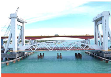
New Pamban Bridge, Rameswaram - operating with structural wire ropes
