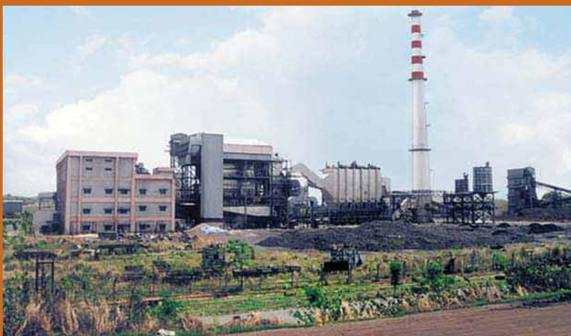
25 MW Thermal Power Plant for captive consumption, Jamshedpur
