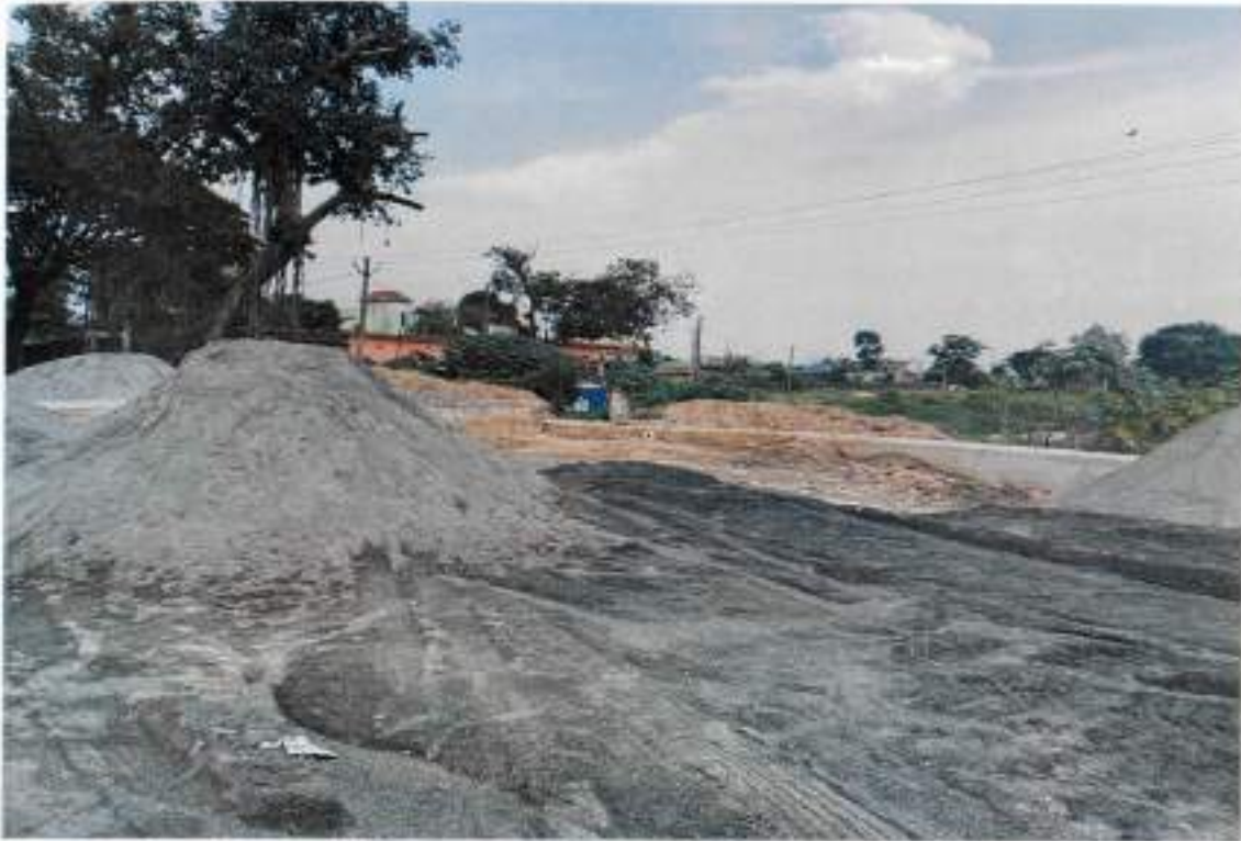
Fig.4: Fly ash use in road making
