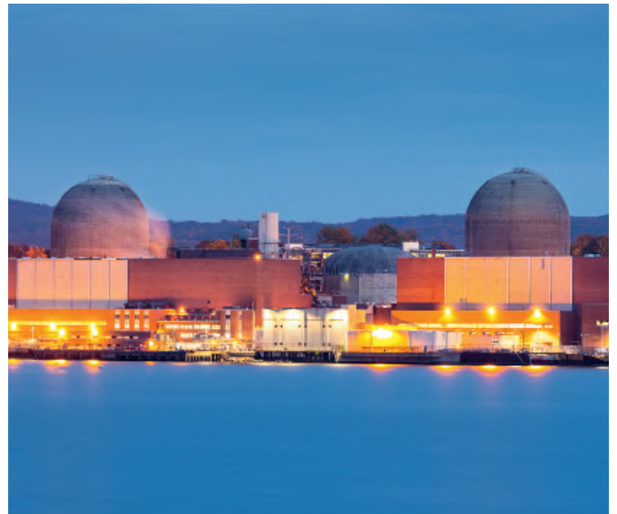
Nuclear Power Plant
