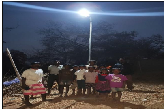
Solar Street Light
